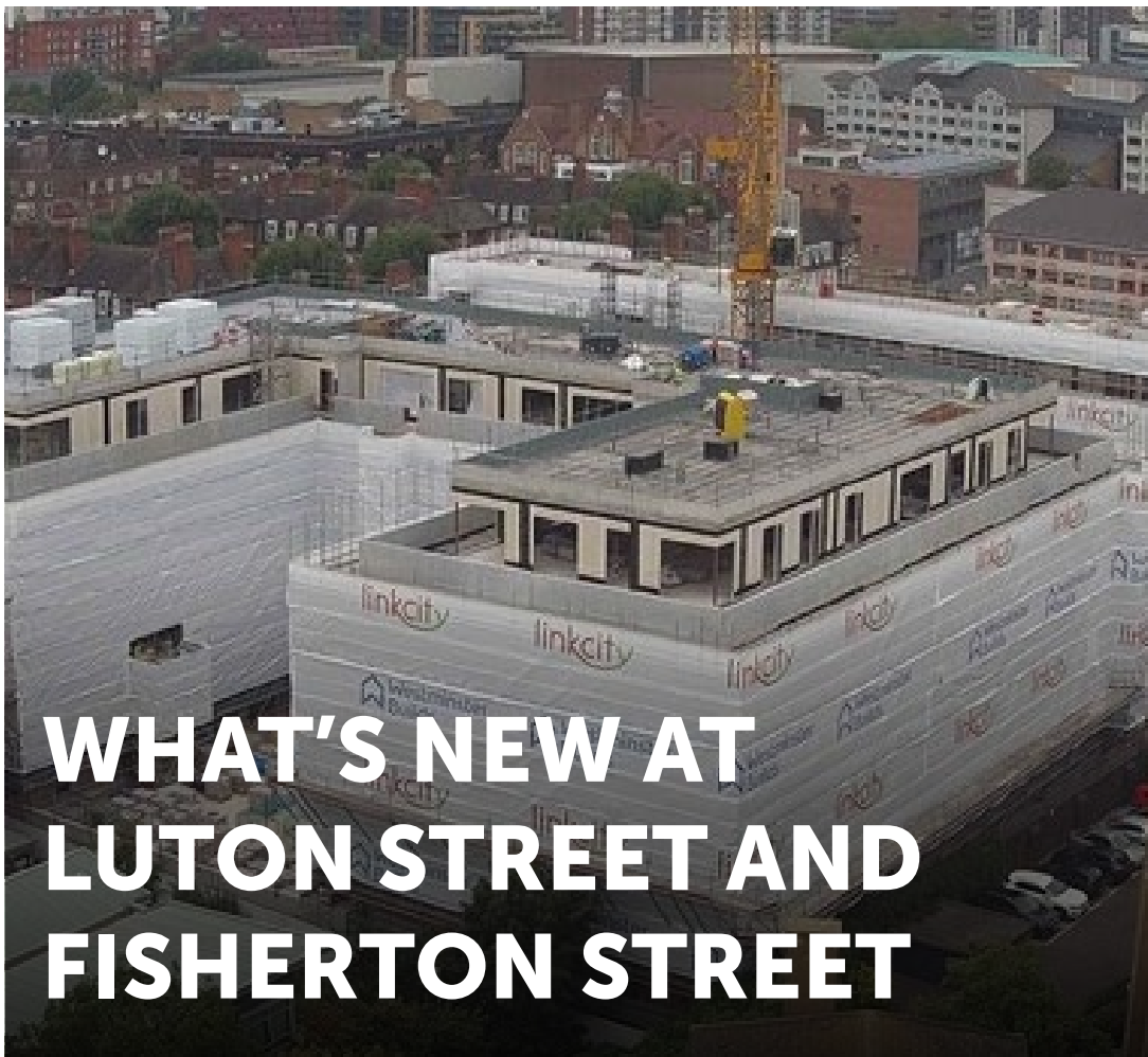
A progress picture of Luton Street
