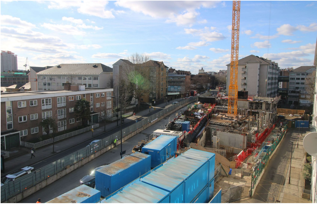
Progress on site at Lisson Arches
