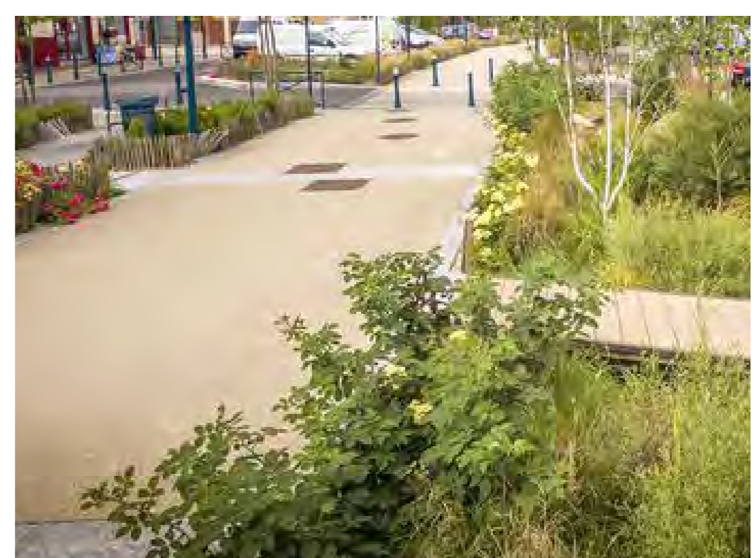
Resurfacing to promote traffic calming
