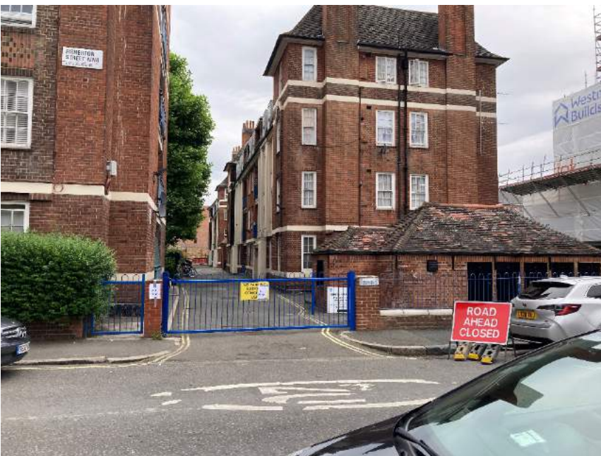
Figure 12: Fisherton Street Conservation Area (i)
