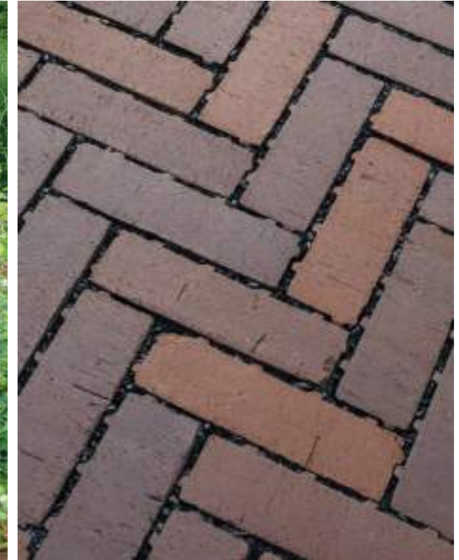
Permeable paving system with drain joint
