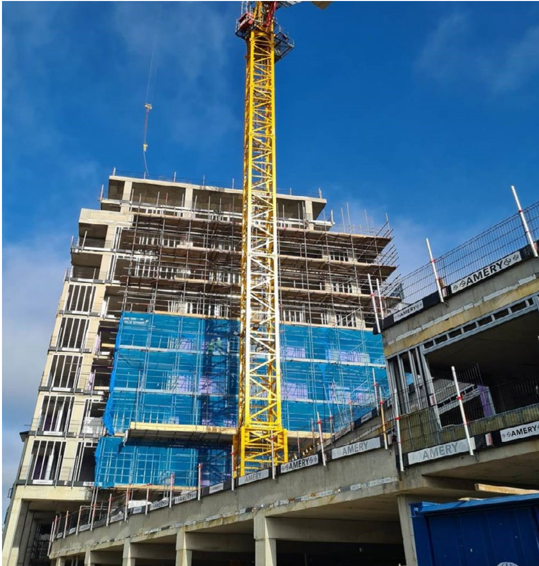
Progress on site at Lisson Arches
