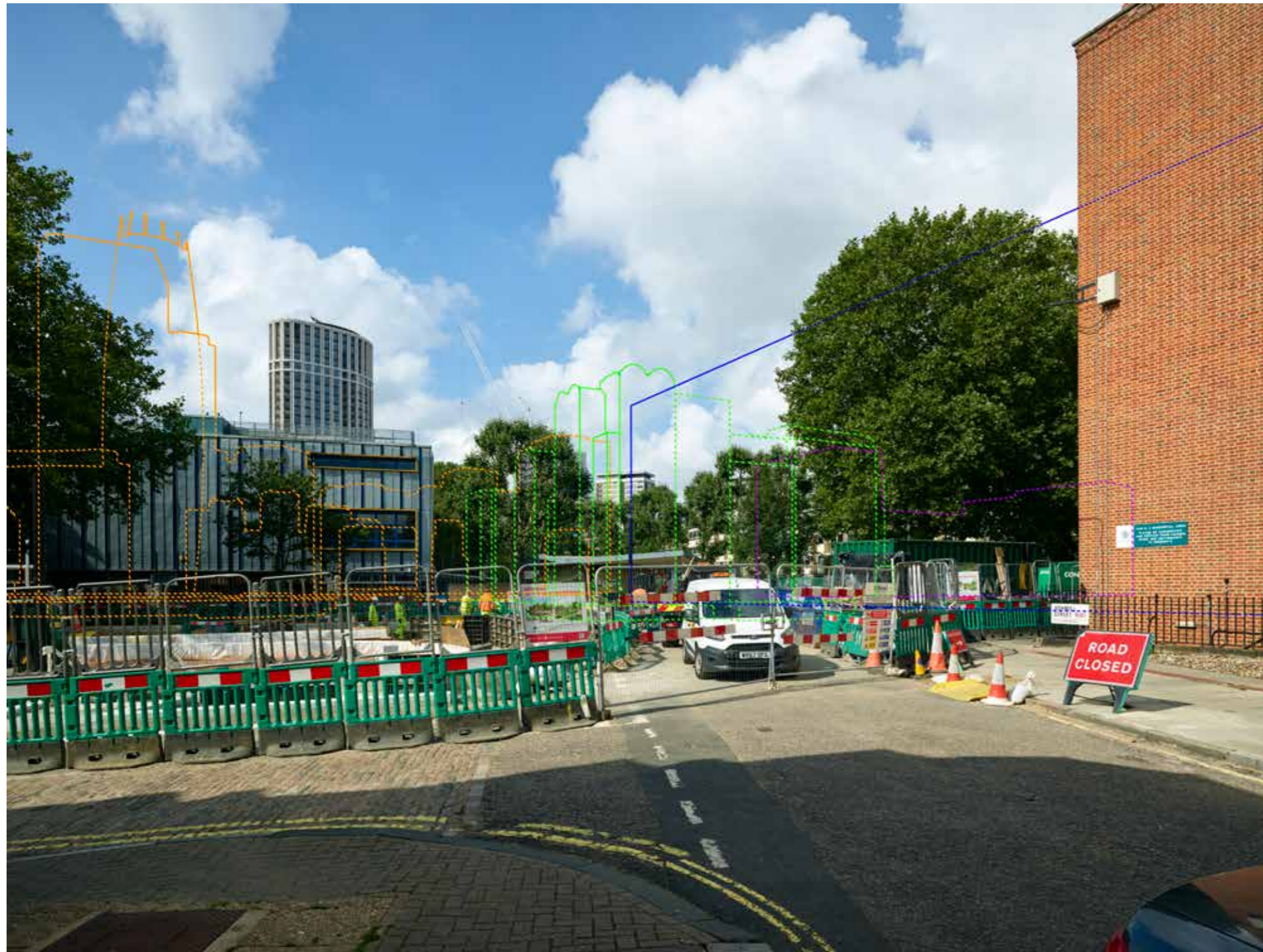
RV 8. Ashmill Street, junction with Ranston Street - Cumulative
