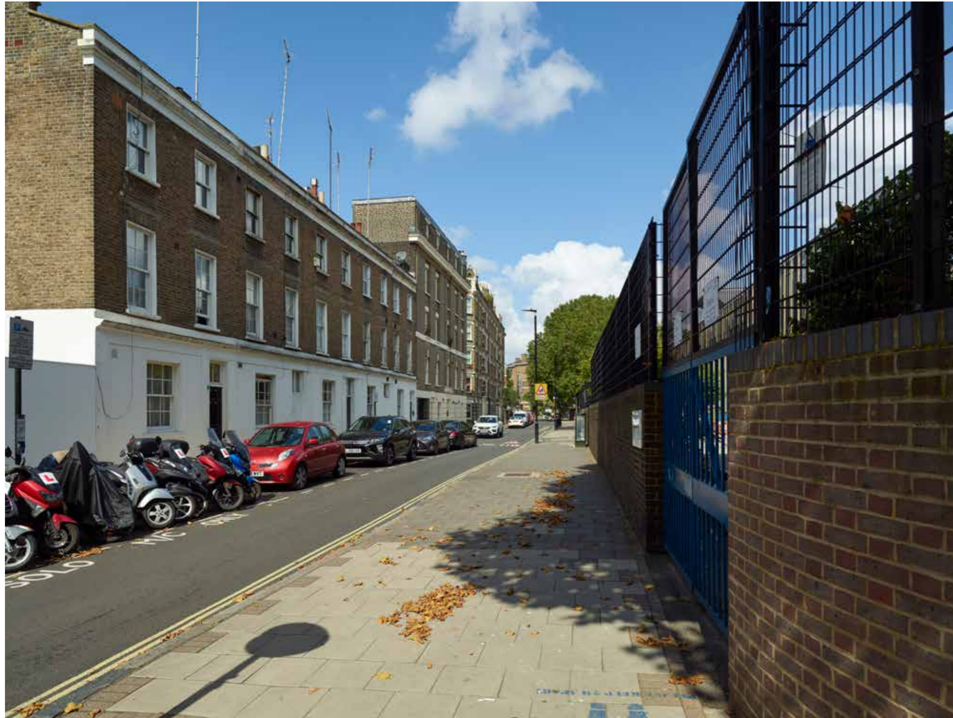
RV 6. Penfold Street, junction with Bell Street - Baseline
