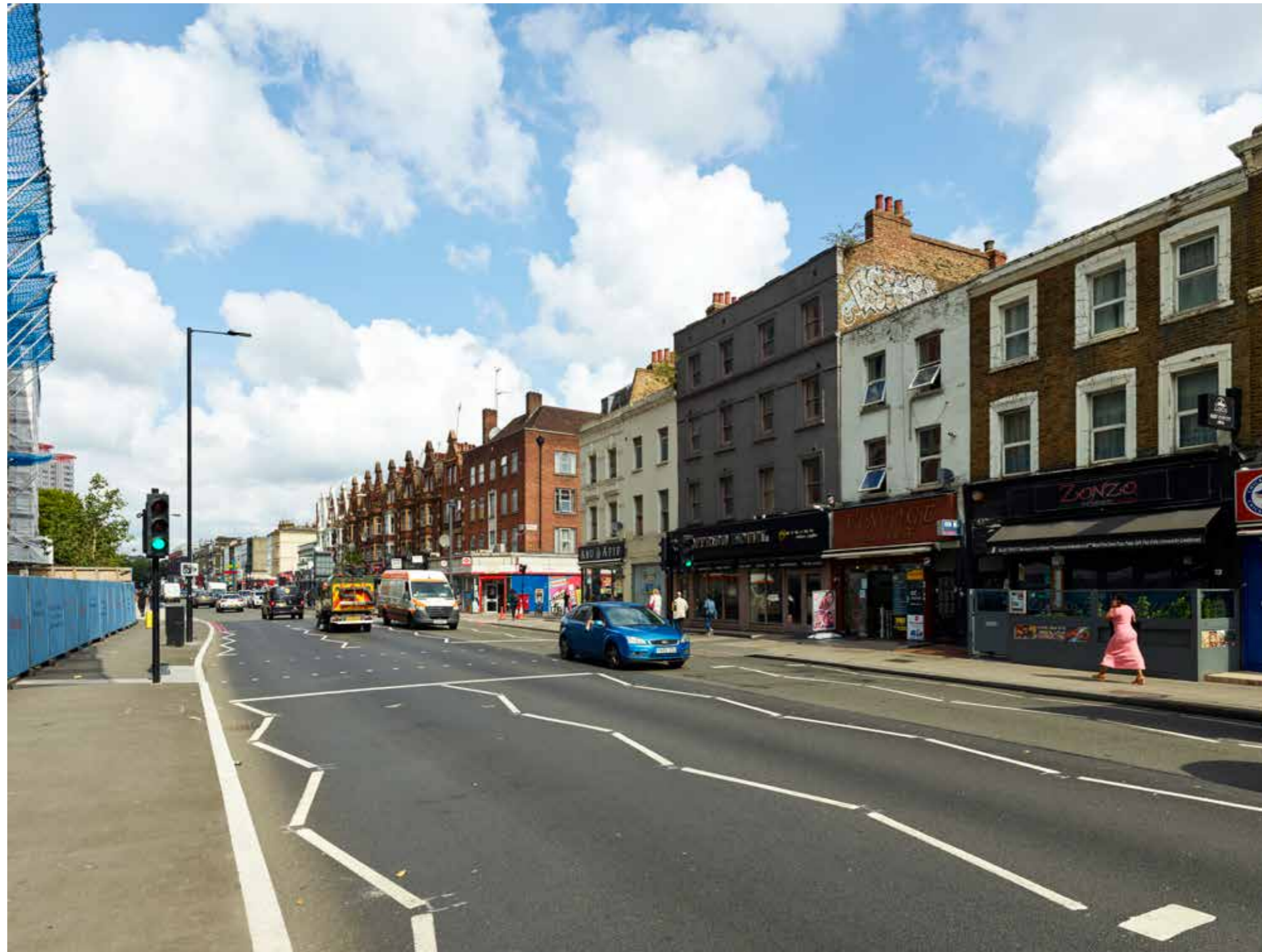
RV 5. Edgware Road, junction with Broadley Street - Baseline
